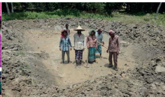
Digging for making water reservoir at crop field
