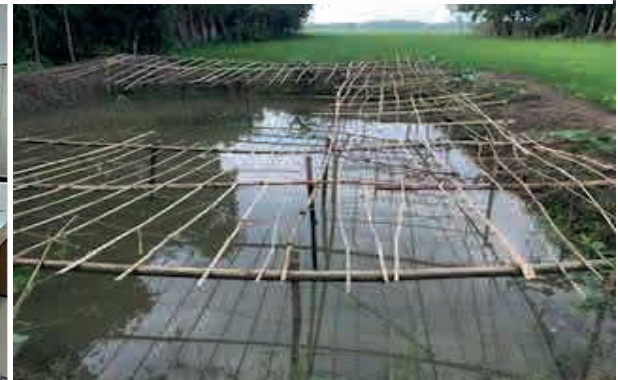
Fencing to grow vegetables on reservoir & to protect children
